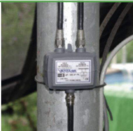
DS 2/1 PL switch connected to the C and Ku-band LNB's of a 10-foot dish
